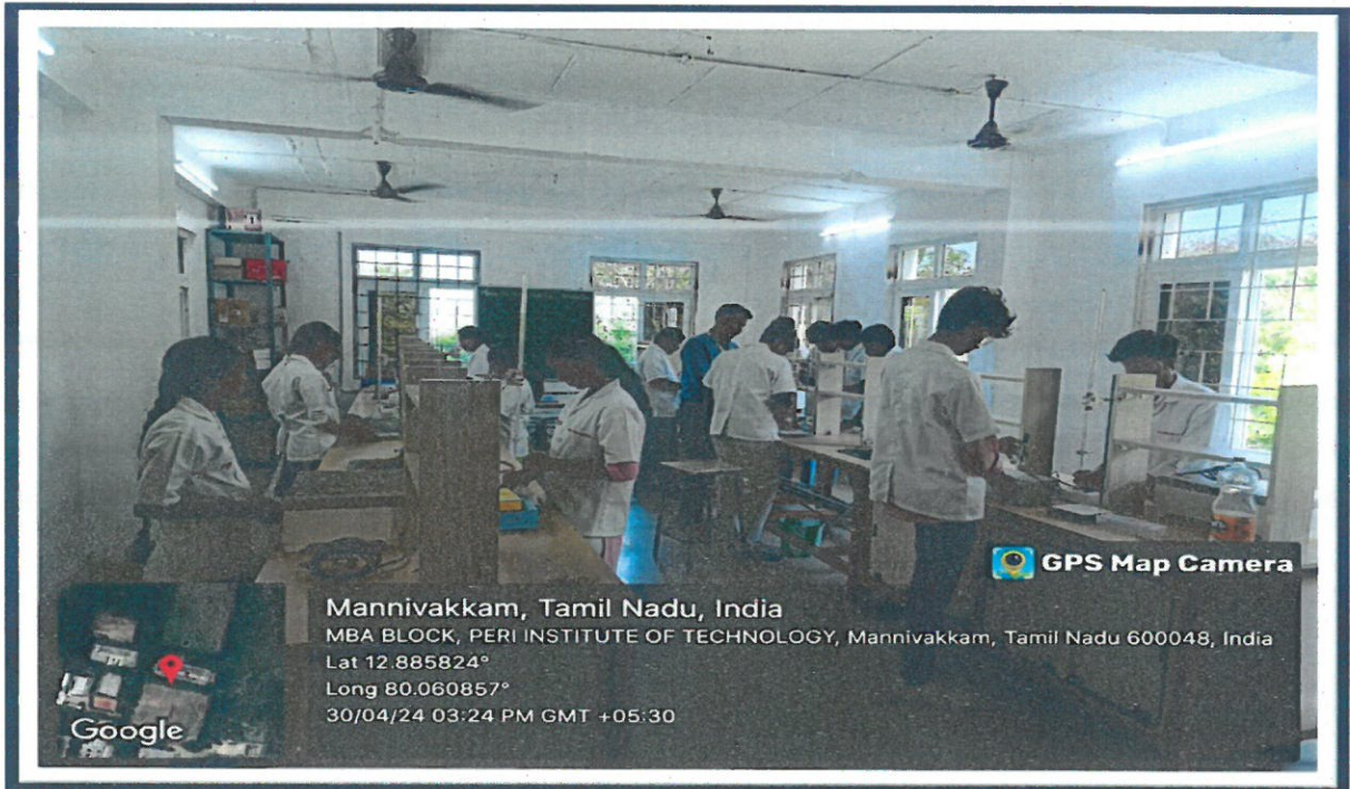
LED Tube Lights at Engineering Chemistry Laboratories
